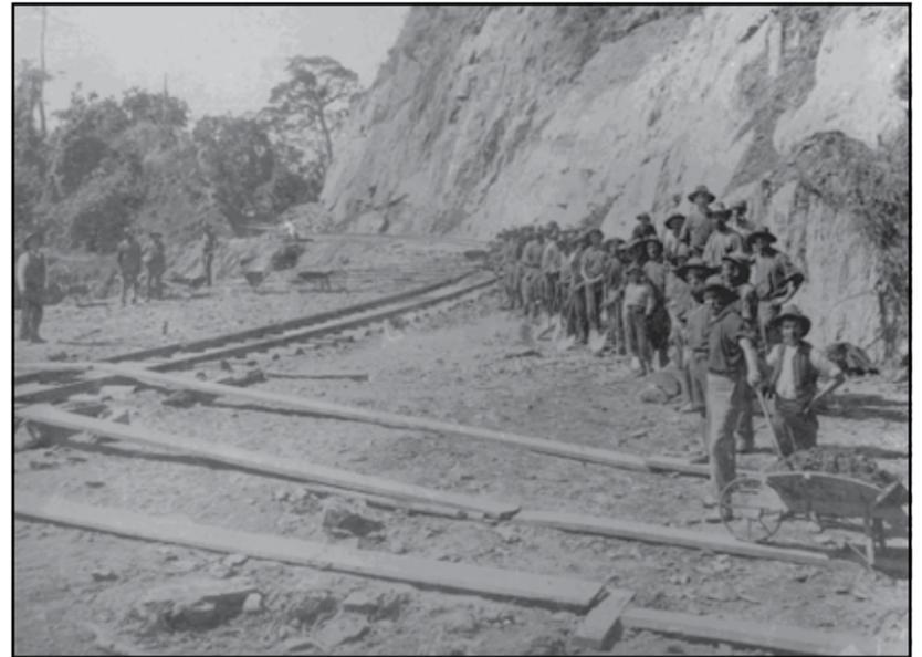
Workers removing overburden near No. 11 tunnel
