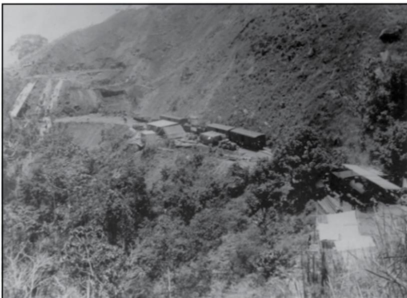
*Washout at Kuranda side of No. 10 tunnel*
